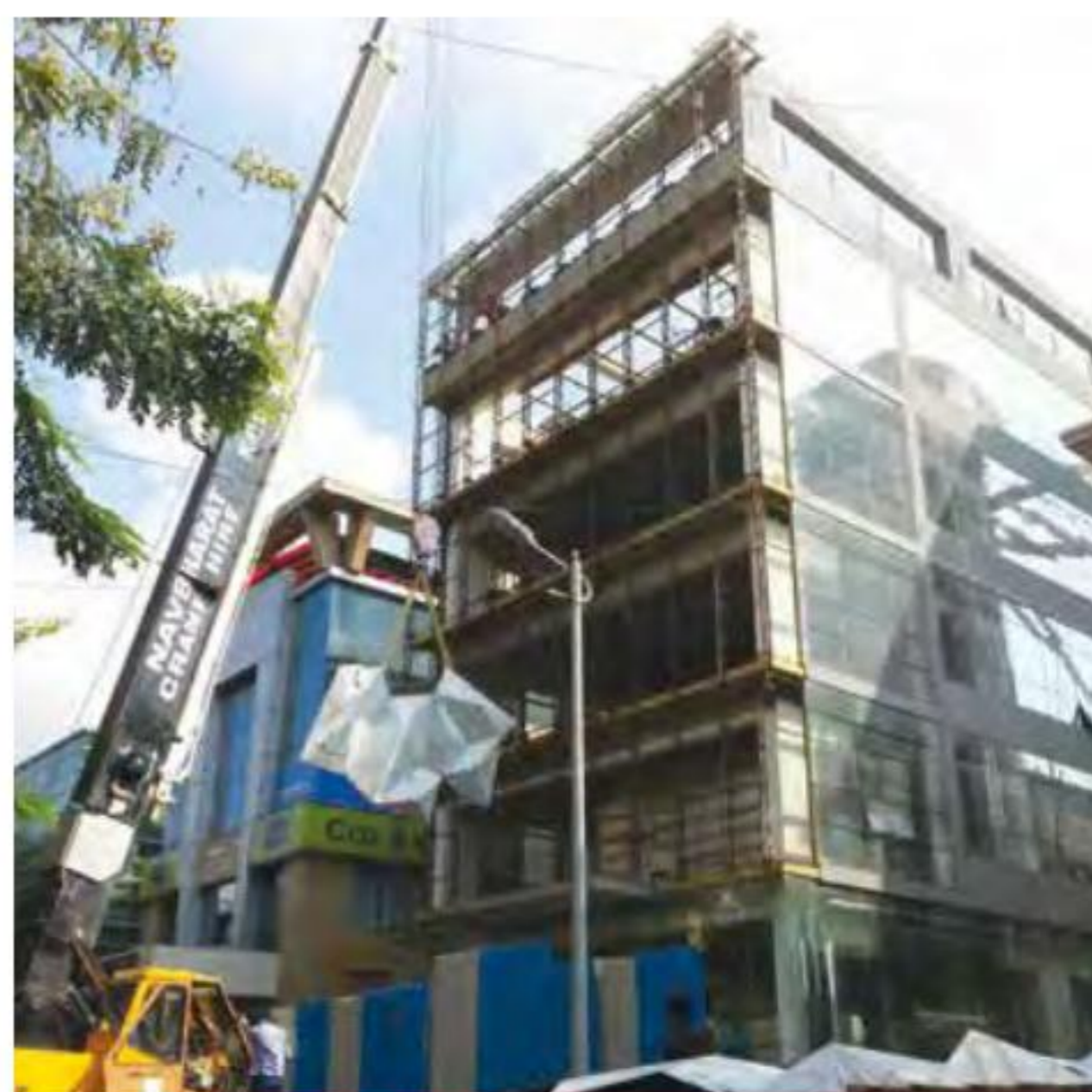
Red cluster assembly work in progress
