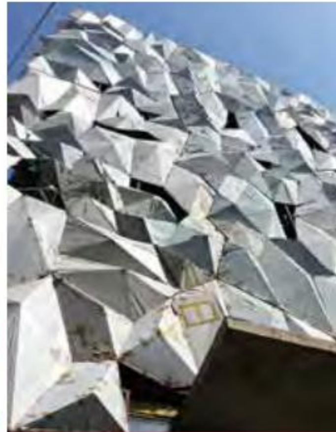
The facade before removing protective film
