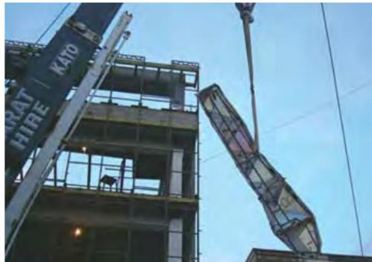
Red 1st Cluster of 6 pieces taken for installation
