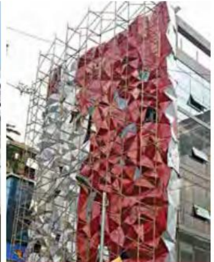
During removal of protective film
