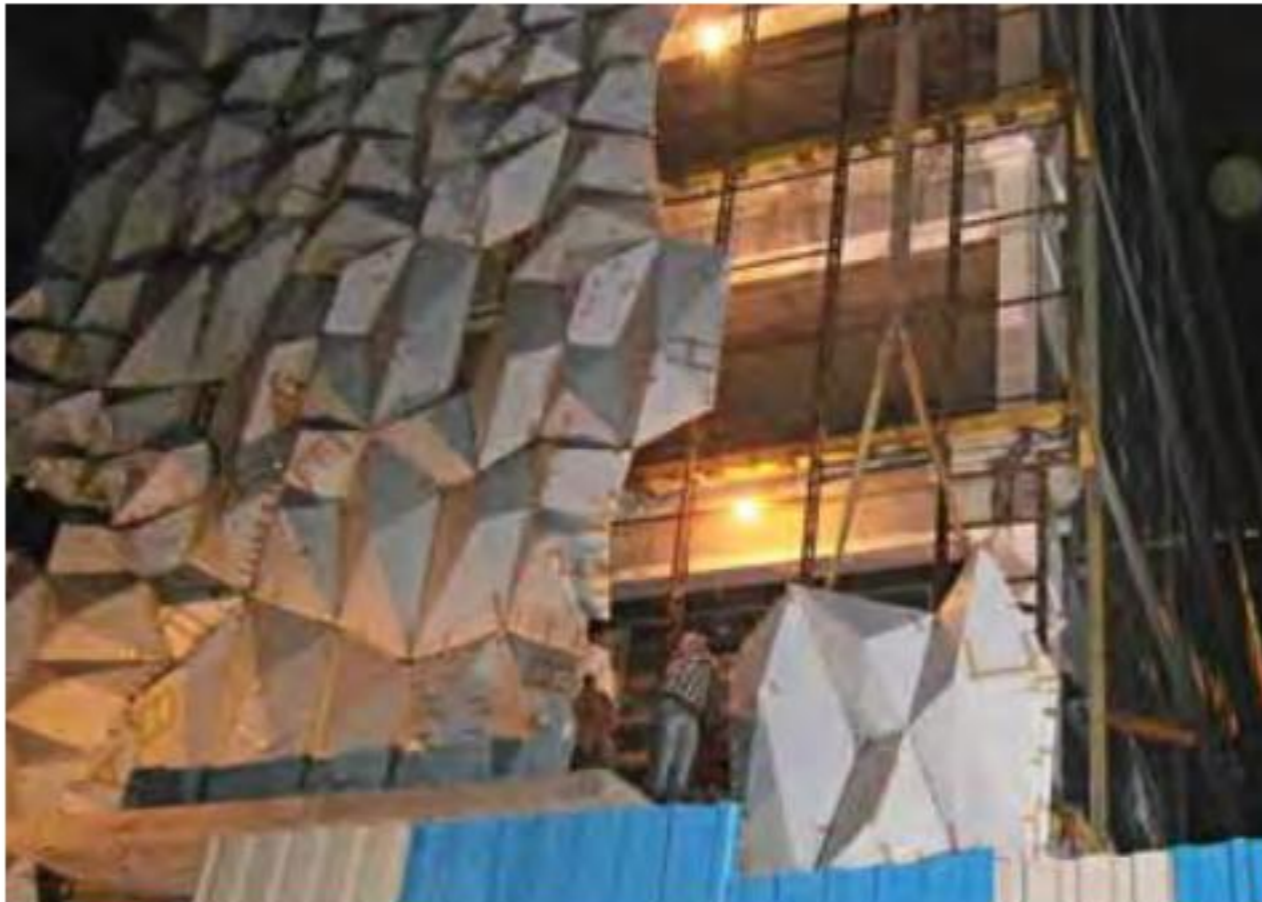
Cluster assembly work progressing at night
